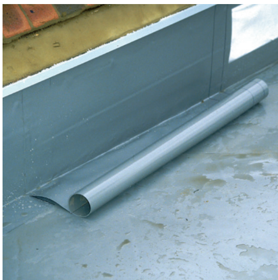
Fig. 1: Edge restraint with RENOLIT ALKORPLAN 81170 metalsheet
